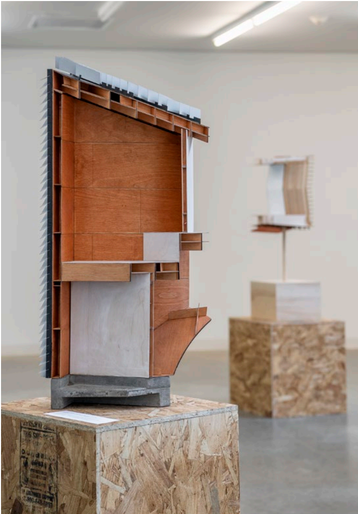
Fremd Zone Detail Model, 1:16 Detail model demonstrating the construction and assembly logic of the building envelope.
